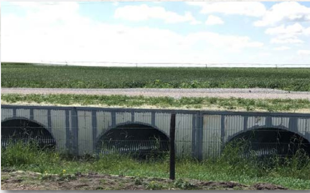
Ohiowa, Nebraska: Triple 71" X 47" Corrugated Steel Pipe Arch on 45 degree skew cut. Headwall reinforced with steel channel and dead man anchors.
