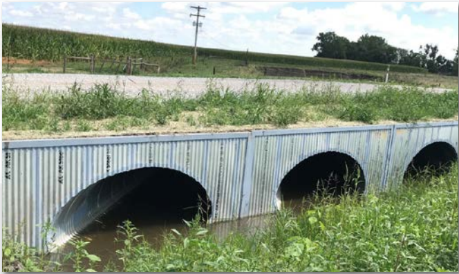
Ohiowa, Nebraska: Triple 71" X 47" Corrugated Steel Pipe Arch on 45 degree skew cut. Headwall reinforced with steel channel and dead man anchors.
