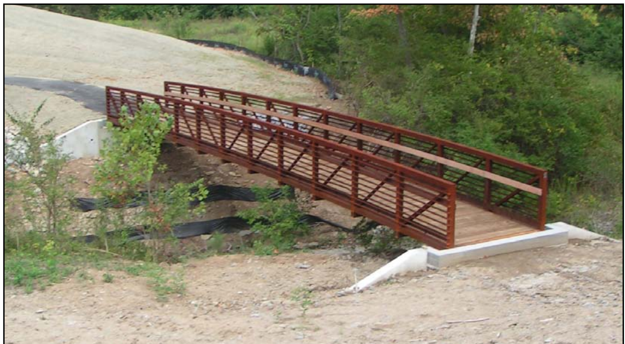
Precast Abutment System installed (Colerain, OH) – Readily available materials and precast pieces means quick installation and overall faster project cycles
