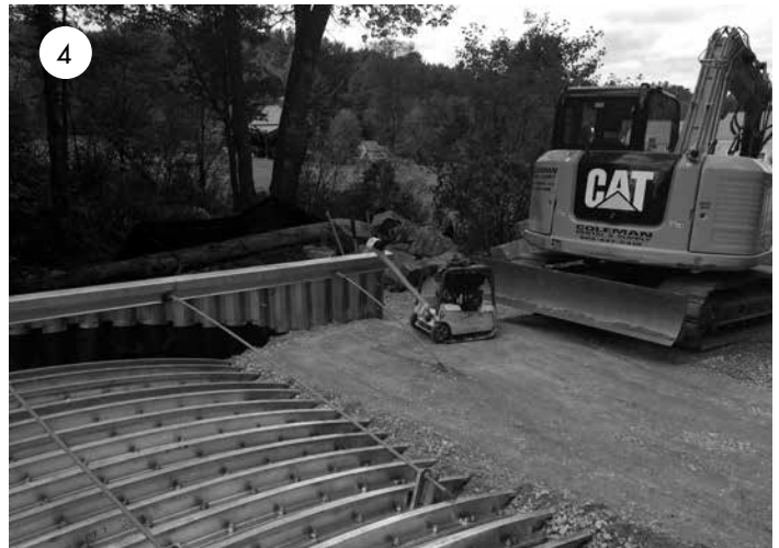
Small tracked vehicles are okay once sufficient cover is placed and compacted.
