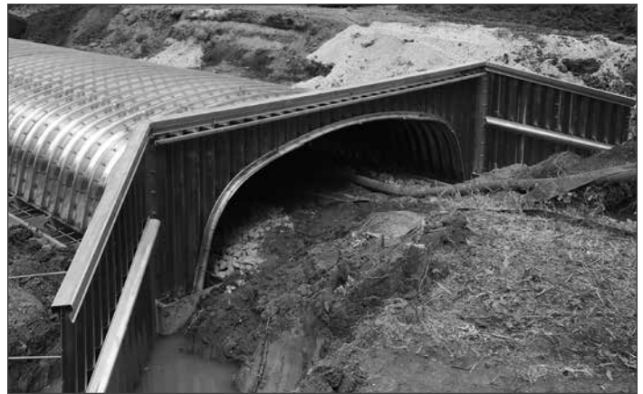
ALBC with headwall and wingwalls.
