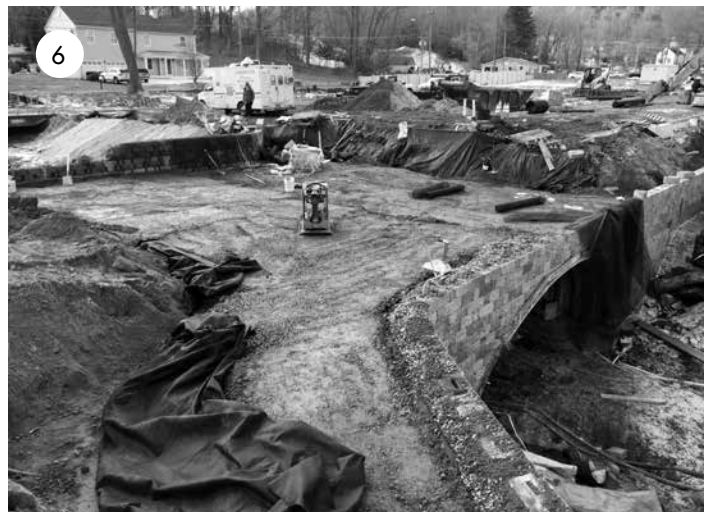
Compact material with a vibratory plate compactor.
