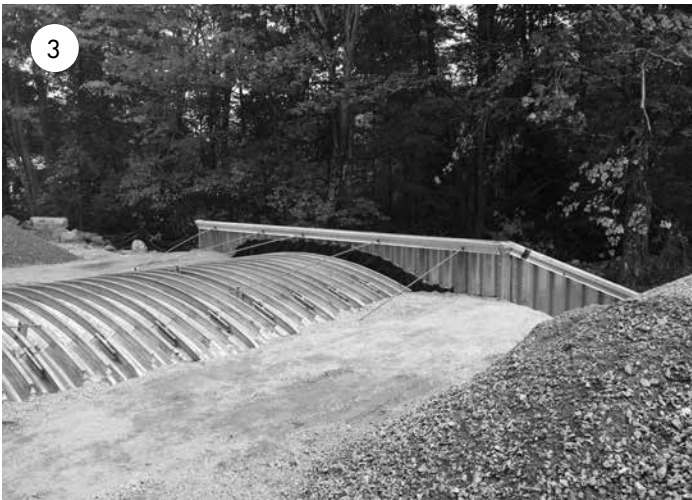
Granular material placed in balanced manner.
