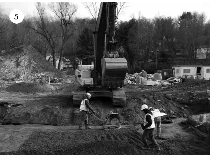
Backfill material is placed and spread from a distance with an excavator.
